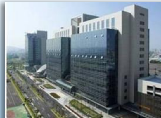
Headquarters (Hsinchu Tai Yuen Hi-Tech Industrial Park, Taiwan)
