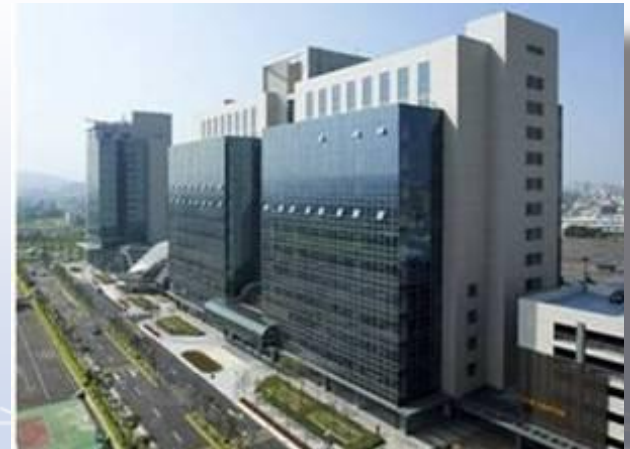
Head office (Hsinchu Tai Yuen Hi-Tech Industrial Park,Taiwan)
