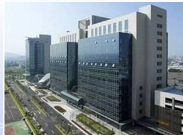
Head office (Hsinchu Tai Yuen Hi-Tech Industrial Park, Taiwan)
